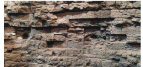
Photo of AUREX® 30SR lance port area after 200 heats with 6-8" remaining lining thickness
