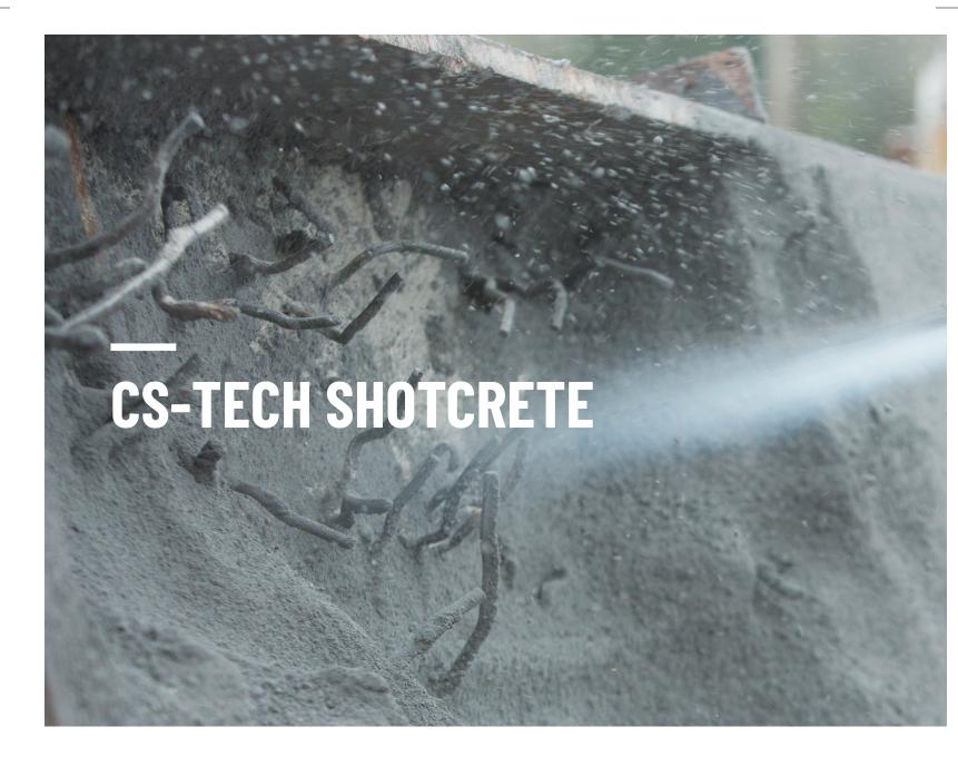
HWI is proud to introduce CS-TECH, a family of cement-free colloidal silica (CS) monolithics. These materials use a colloidal silica liquid that acts as the bond phase in the matrix. This allows for better adhesion to existing refractory linings than other no-cement formulations, while offering the traditional benefits of no-cement products.
