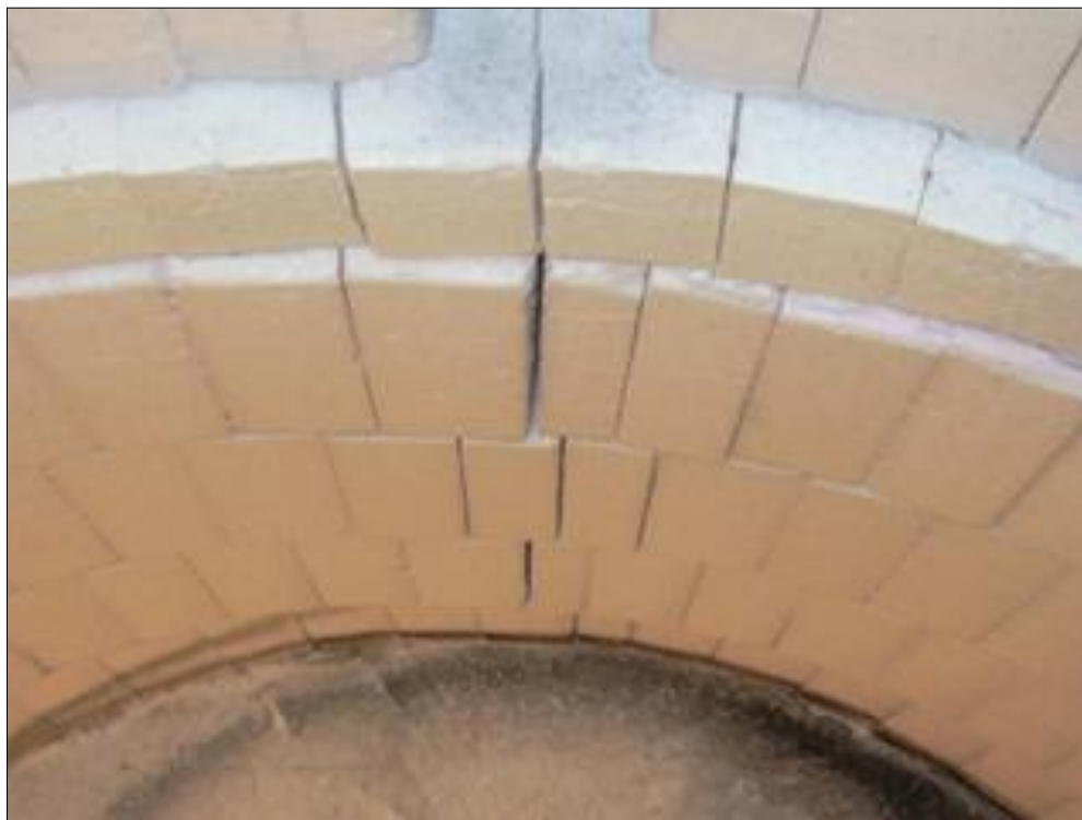
Figure 7: Flattening of bricks along top center of thermal reactor.
